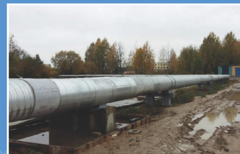
«Boiler on Sosnovaya Str. in Kostyukovich», 1 stage of construction. Off-site heat supply networks 2Du500 mm, above-ground laying.
