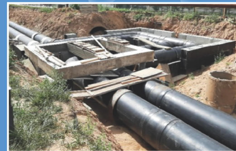
«Reconstruction of a heating main using Pitrub TM-01 in the section from TK-0118 to a point in the area of TK-0127 on the Ulyanovskaya Str. in Bobruisk.» 2Du800 mm, U-shaped compensator.
