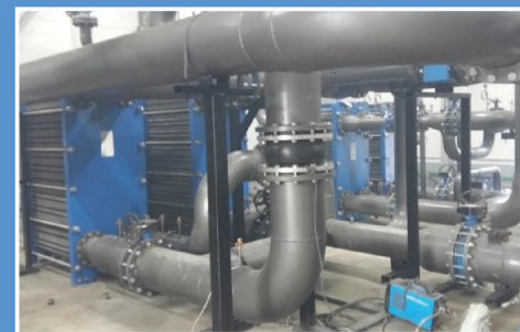
«Construction of a heating network in the city in Borisov from UT6 in the area of the boiler house on Brothers Vainrubov Str. to the district of heat supply of boiler room No. 5 on Serebrennikov Str. with the construction of the central heating substation,» central heating substation, installation of equipment.
